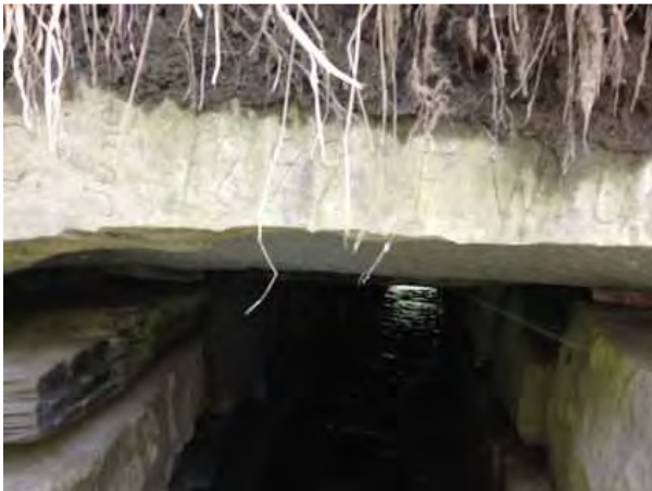
This stone culvert's lintel stone bears the date June 1899 along with the initials of the individuals who worked on the road crew and most likely constructed the culvert. (Image property of VTrans)
